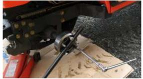
H. Reinstall the wheel & install the & torque the new gold nuts to 65 ft. lbs for the rear wheels.
